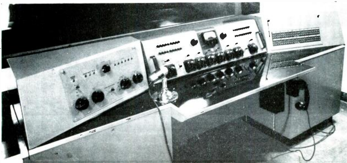
Fig. 5. In Studios C and D, a standard RCA 76-C consolette is used in conjunction with auxiliary custom-built side turrets (jack bay at right—and sound effect filters, echo controls, cue selector and supervisory lights at left). Space is provided for turntables at each side of the operator's position.
