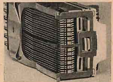
New relays must be able to operate one billion times—equal to once-a-second for 30 years. Employing a sound recorder as a precision vibrator, Bell scientists learned to evaluate the effect of sideways motion on relay life. Such rubbing motion is limited to one-thousandth of an inch in the new relays.
