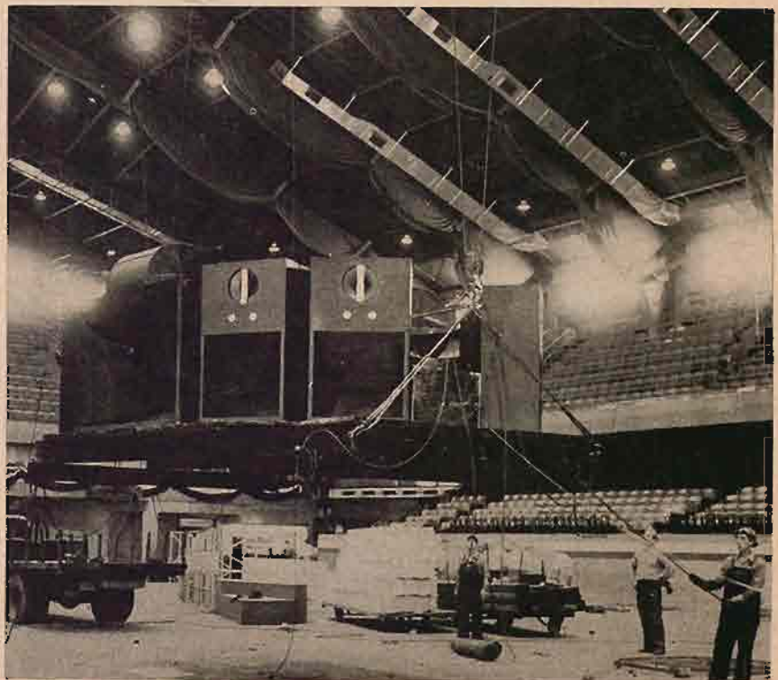
Fig. 6 The reproducer gondola just before hoisting to its operating position.
