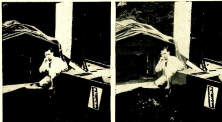
Fig. 2. Another stereo pair. Mr. Green in the throes of installing the speaker system in the structure built just to house it on the roof. This in one installation where the user won't be changing the balance between high- and low-frequency units very often.
