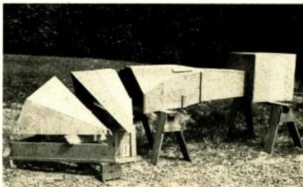
Fig. 3. By constructing the horn in sections, it is possible to handle it without the aid of a crane.
