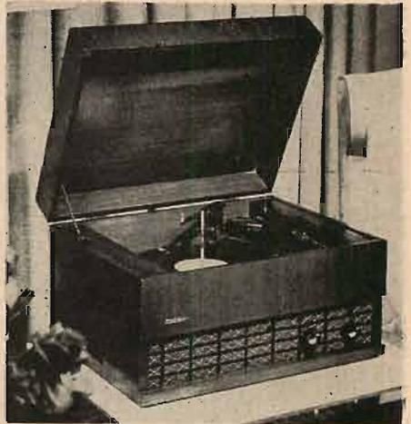
an audio response of 50 to 12,500 cps. Changer is the Webcor Type 121 which plays records of all sizes and speeds automatically, and which is equipped with automatic shut-off. A five-tube amplifier affords five watts output with low distortion. Webcor-Chicago Corporation, Chicago, Ill.
