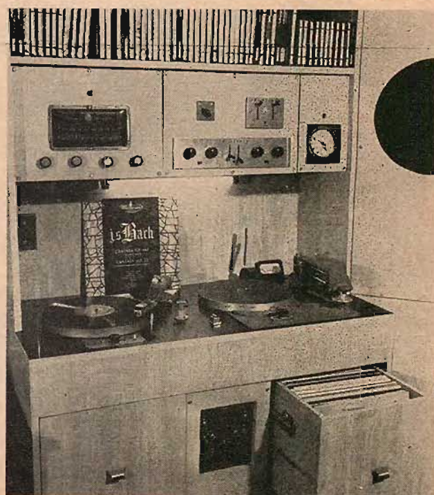
Fig. 7. A close-up of the main console. Note timing clock and switch and patch panel below the table.
