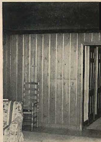
Fig. 5. This photo shows how the entire installation is covered by the vertically sliding panels when it is not in use.
