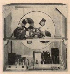
Fig. 11. The Allen Gyrophonic Projector-a device which introduces a vibrato by mechanico-acoustic means.
