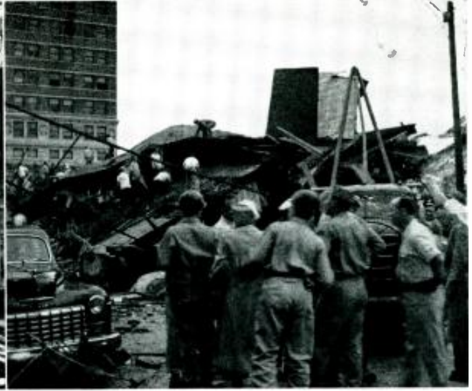
This pitiful heap of rubbish was the five-story R. T. Dennis Company, furniture dealers. More than twenty-four persons died here. The author supplied 115 articles on tornado damage to magazines.
