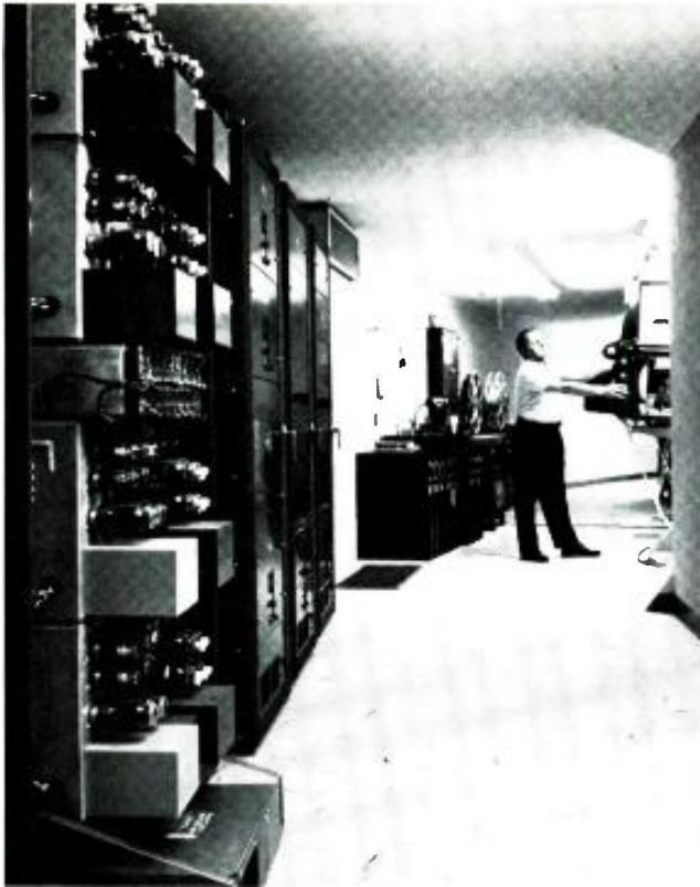
Figure 1. The Century 21 theater in San Jose, California features four racks of a six-channel magnetic theater sound system. This installation has the older vacuum-tube model, which has since been replaced by solid-state units.
