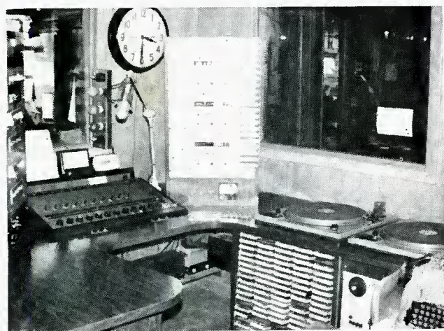
Figure 4. An over-all view of the finished control room. Turntables are installed for the convenience of handling Sunday morning religious programs and specialty items, not normally for music.
