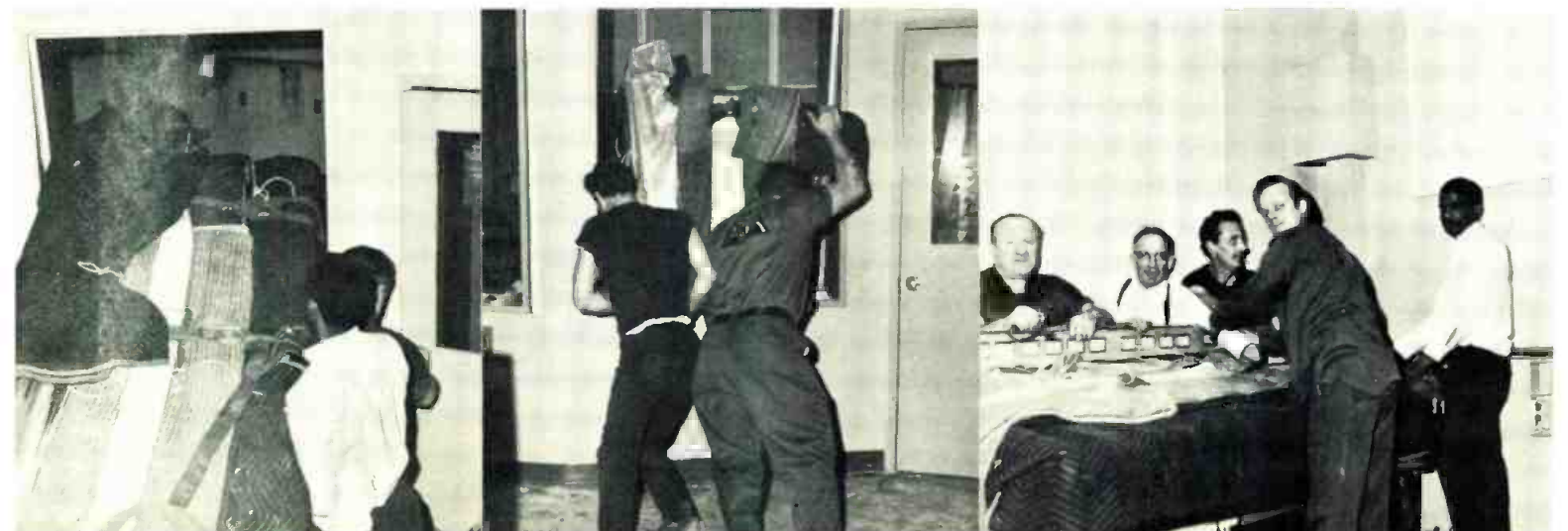
The control room door was much too small, so out came a double window into which the console just fit. Pushing and heaving gets it through and into position in the room.
