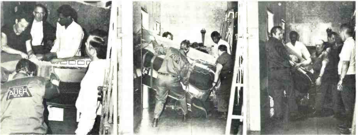
Cables and other rigging are attached from the bottom of the elevator to the console. Slowly the elevator starts to rise, pulling almost nine feet and one ton of electronic gear slowly into the elevator shaft.
