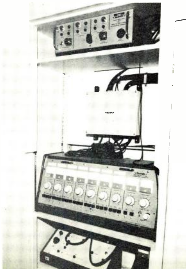
Figure 2. The equipment used to drive the auditorium sound-reinforcement system, and for the r.f. amplifier loop used for simultaneous language translation in the auditorium.
