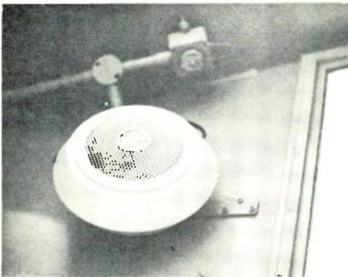
Figure 3. One of the many loudspeakers scattered throughout the ship, and another instance for which the generic word for sound reinforcement systems in Great Britain is Tannoy. These speakers are unobtrusively placed and can be heard clearly when required, with light background music coming from them most of the time.
