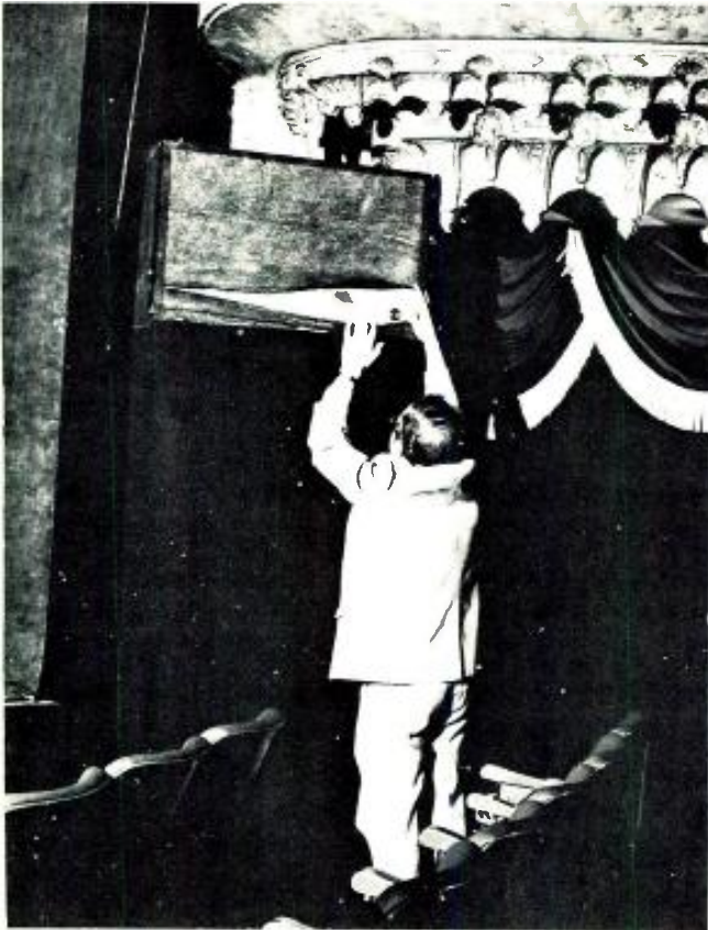
Figure 2. Two more Sentry IIs deliver all the sound from the stage performers. They are installed just a few feet from the proscenium, one on each side.
