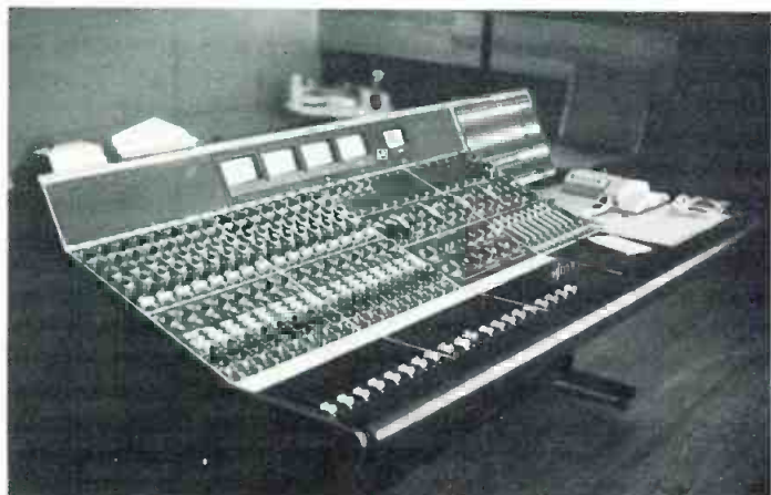
The other control room has a (more or less) stock Neve console that was installed with a great rapidity and without a hitch. It has 16 channels in, and as many out, and is currently being modified.
