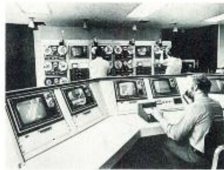
Figure 1. This is the origination studio of Trans-World Communications. Each of the seven cities in which the company operates has an identical control point which transmits current motion pictures to all the hotels hooked to the system. The "mini-computer" in the foreground transmits the selected features to the guest's room within 33 milliseconds of receiving the order.
