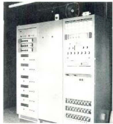
Located in the main control room, the fan-cooled control console incorporates an automatic lighted relay speaker network crossover (bottom right) for emergency transfer of speakers without dispersion loss in case of amplifier failure.
