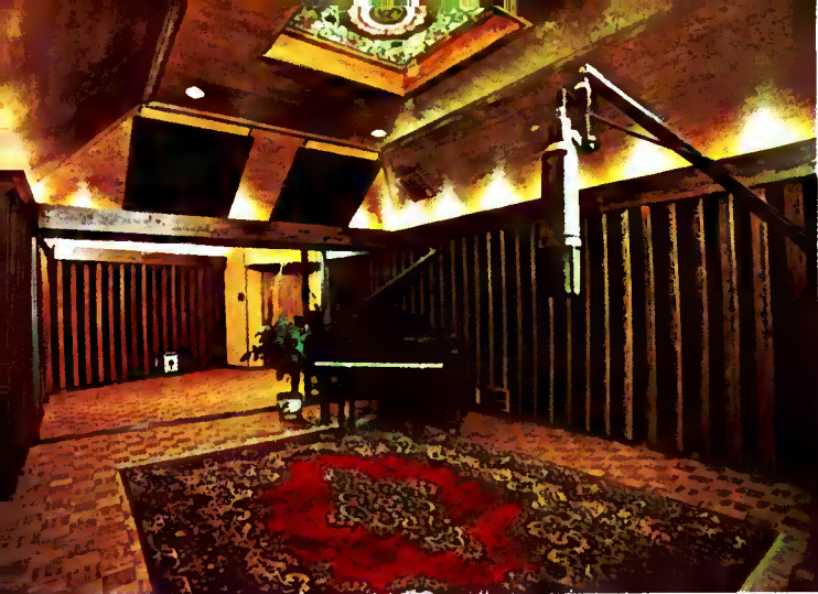
Golden Age Recorders in Culver City, California. This studio features a modular diffuser-slat design to optimize room ambience and increase reverberant field homogeneity. Bass absorption is accomplished by the ceiling resonator cove, and natural light provided by the four-paned acoustical skylight. Acoustic design by Jeff Cooper.
