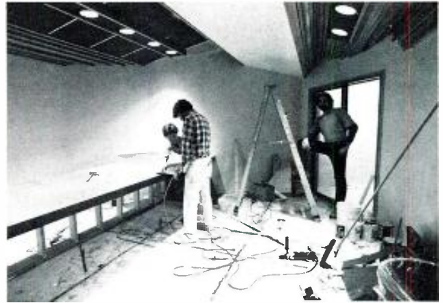
The studio control room under construction.
