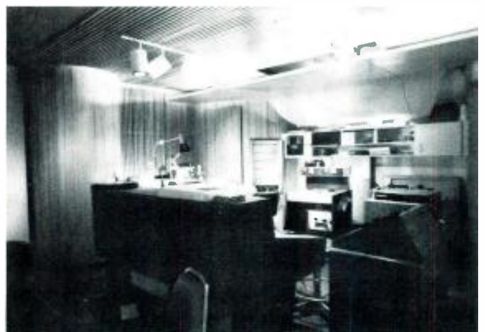
Rear view of new mastering room showing side wall polycylindrical absorber/diffusers, ceiling cloud, and rear wall cabinetry enclosing mastering computer. Grillwork on ceiling and walls is also shown.
