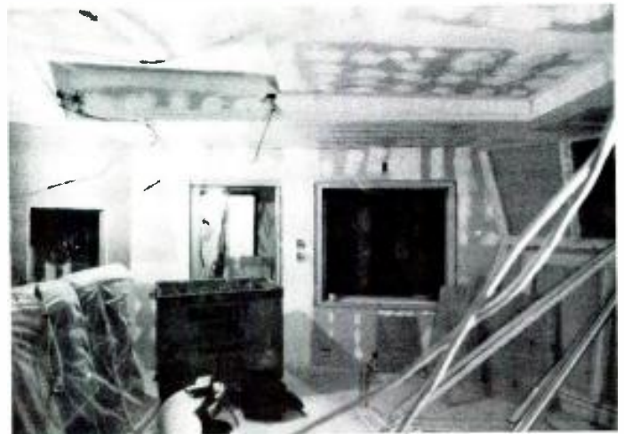
New mix room under construction. On the left is the polycylindrical auxiliary equipment enclosure and the MCI 56 console (wrapped in blankets). On the right is the left monitor enclosure and the vocal room window (through which the MCI console was delivered).
