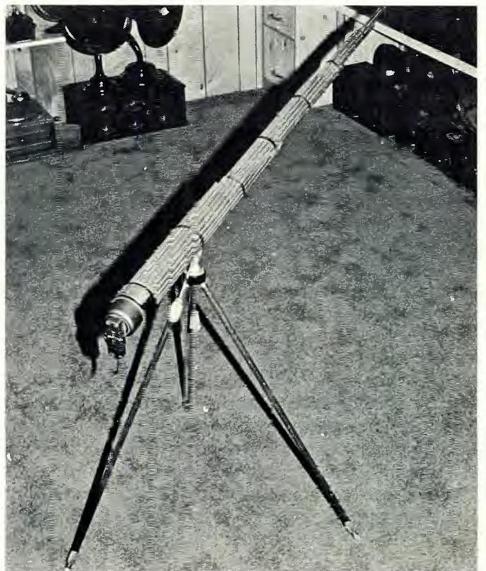
Figure 8. A Western Electric Shotgun microphone, circa 1937.
