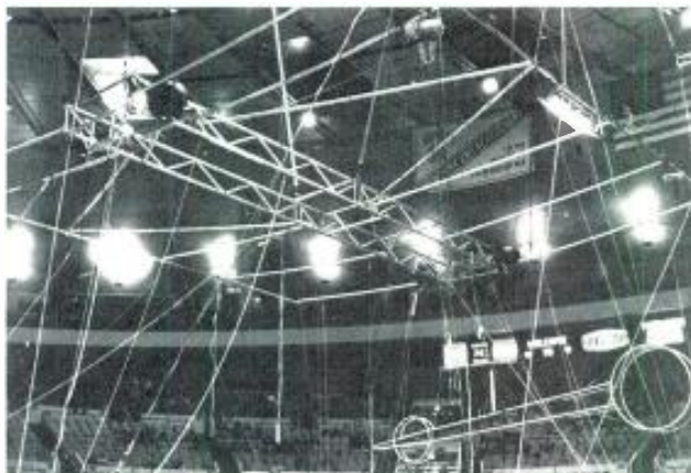
Loudspeaker configuration above Ring Three. (An identical configuration appears above Ring One.)
