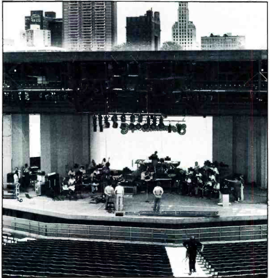
The new amphitheater sound system at Mud Island, featuring speakers in a central cluster arrangement above the stage.
