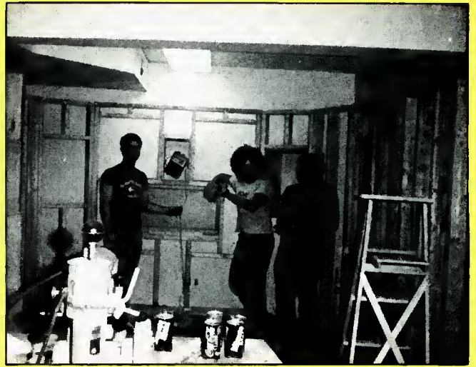
Students building wood formers for walls.
