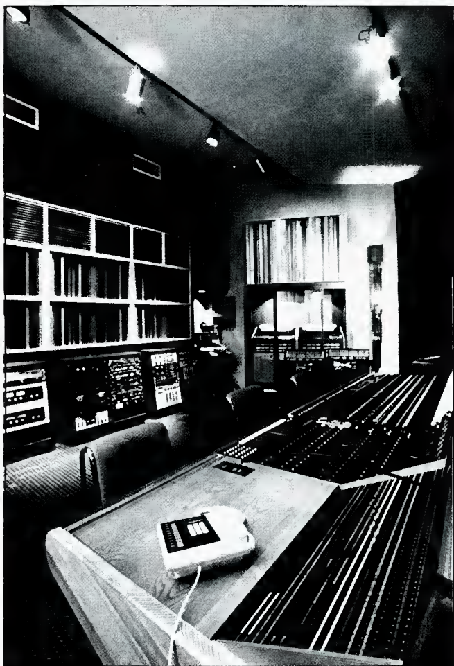
Figure 5B. Rear view of the control room at Master Sound Astoria in the Kaufman Astoria Film Studios, Astoria, NY, showing rear and side RPG diffusors. Acoustical consultant, Charles Bilello Associates.
