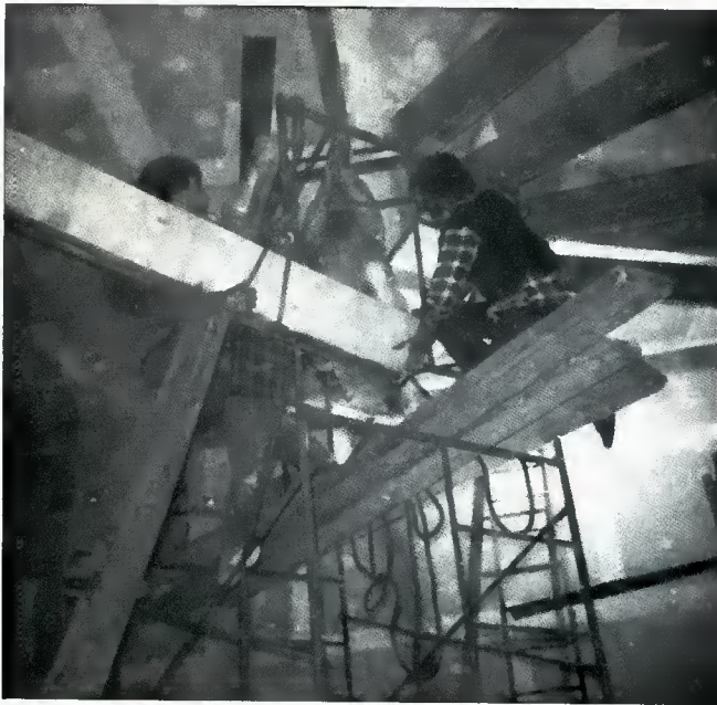
Figure 10. Central convergence, at the ring, of the spider legs.
