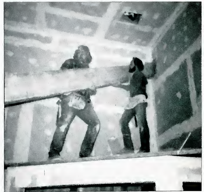
Figure 9. Raising the tripled 2x12s forming the ring's spider legs. The workers are standing on the isolation booth.
