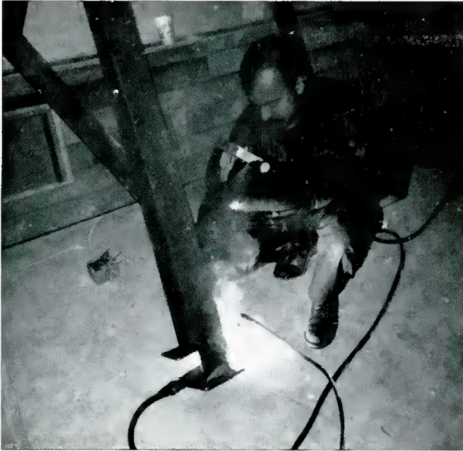
Figure 6. Welding the ring's support structure in studio A.
