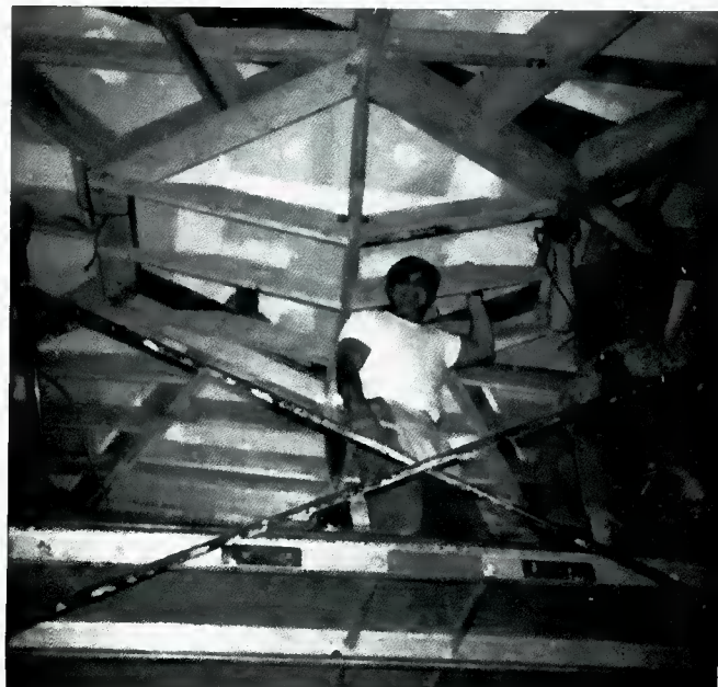
Figure 11. The basic structure of the parabolic reflector frame and radiating legs.
