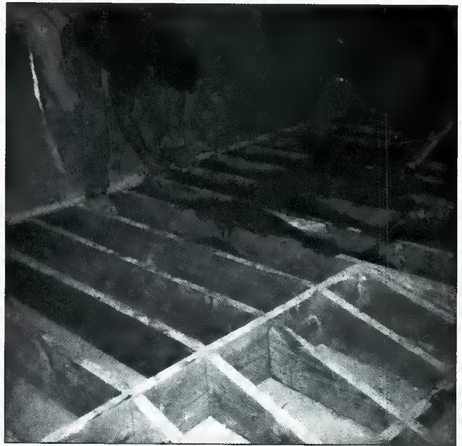
Figure 4. The framing and pouring of concrete for the control room's console platform.
