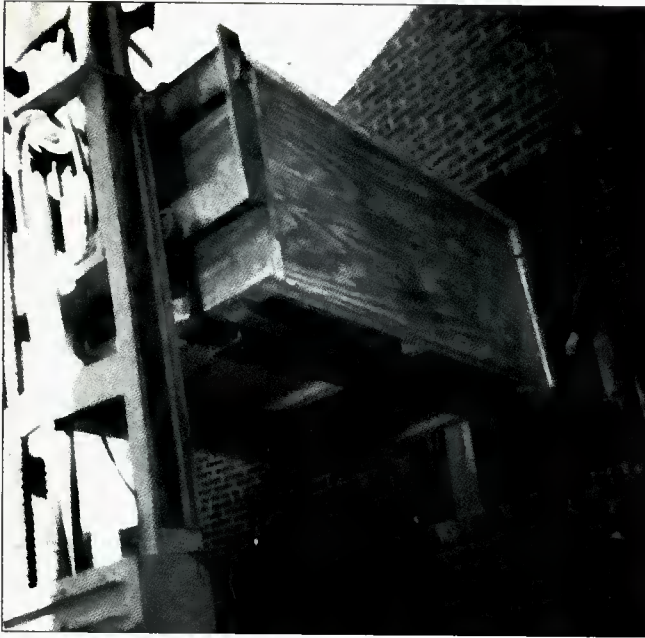
Figure 2. The console being hoisted to the second floor.
