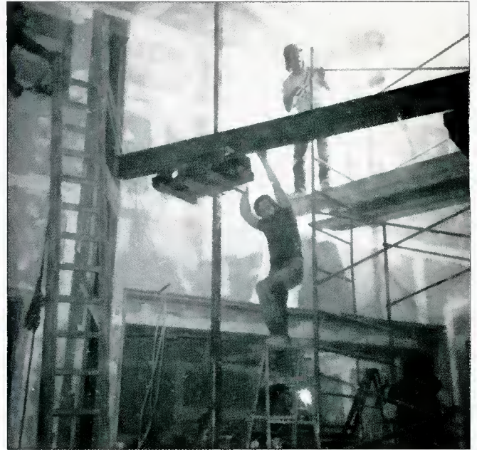
Figure 8. Lifting the "I" beam supports to their positions for welding.
