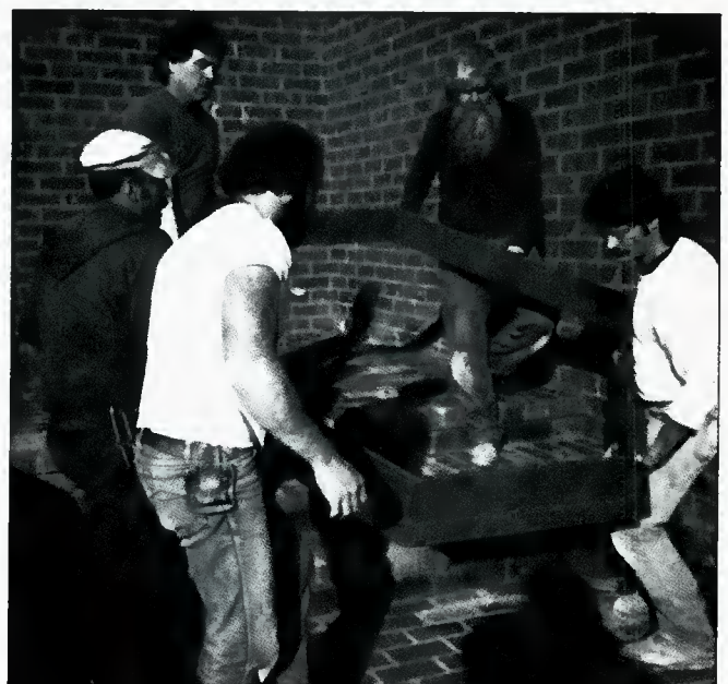
Figure 5. The steel ring for the parabolic reflector. Its approximate weight is 600 lbs.
