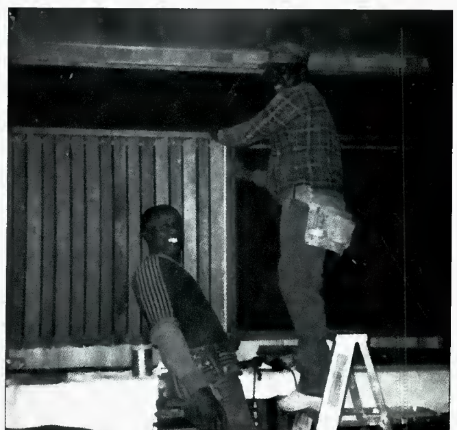
Figure 13. The rear, dead end, of the control room.
