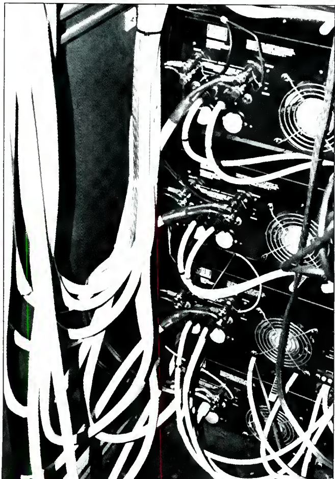
Figure 3. The amplifier rack.
