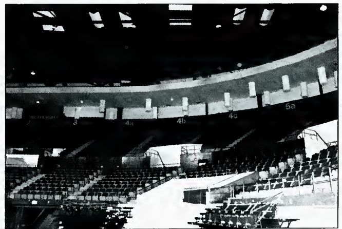
Figure 12. After acoustical modifications. Note the Helmholtz cylinders.
