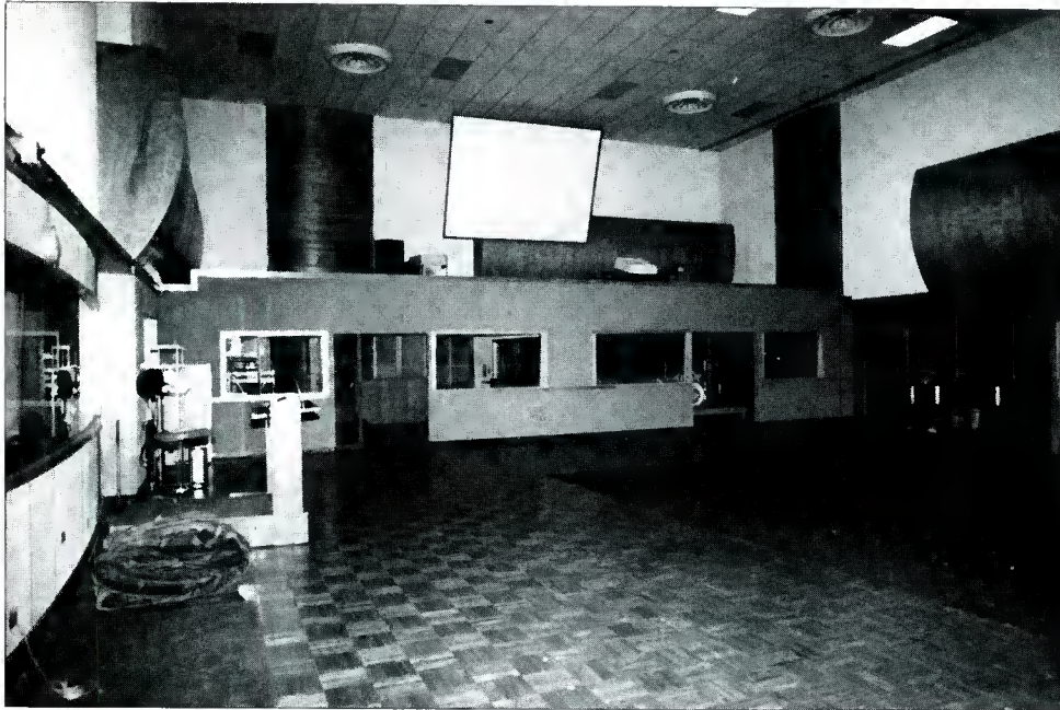
Figure 3. Studio A. Our wide-angle view clearly shows a number of the polys. The ceiling can be moved up or down, according to the exact acoustics needed.
