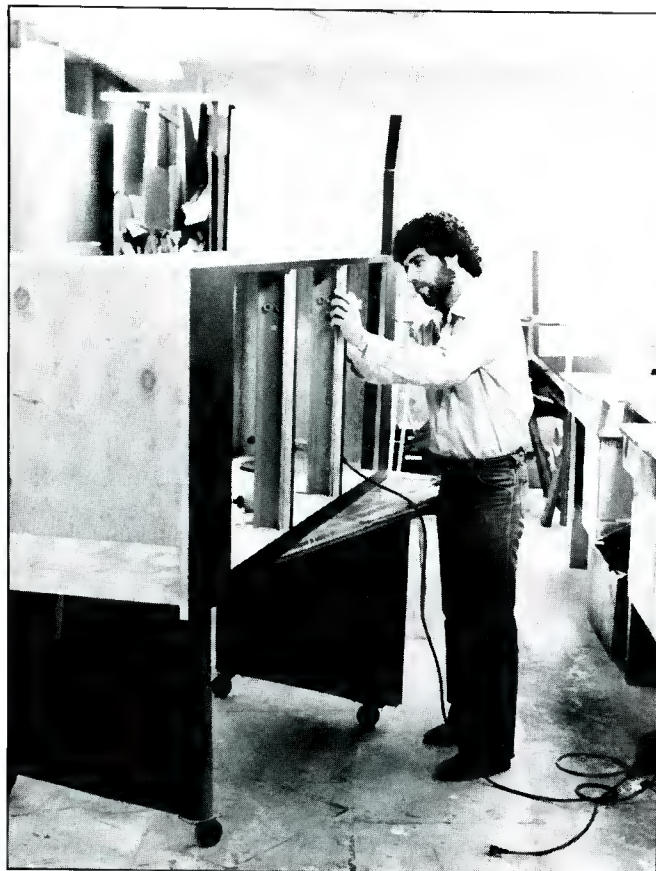
Figure 4. The author is seen finishing the front of the new rack. Steel reinforcement was added to withstand the weight load.
