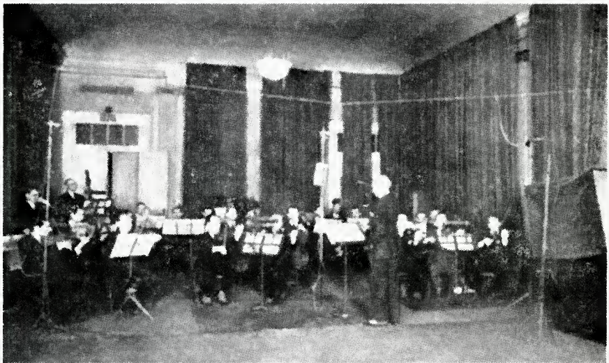
Fig. 1. For the New York demonstrations, the orchestra was in a room two floors above the auditorium. The three microphones were spaced across the room in line with the conductor.
